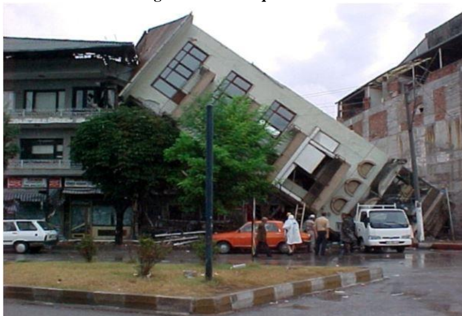
Figure 37 :- Damage in structure due to soil liquefaction
